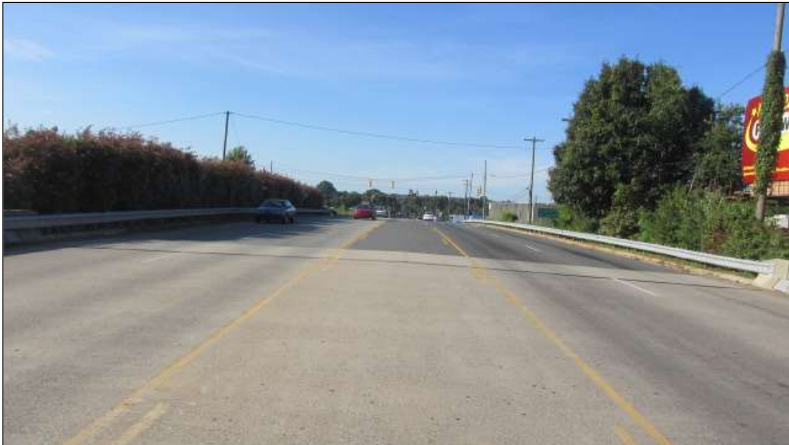
GUARDRAIL LOOKING EAST
