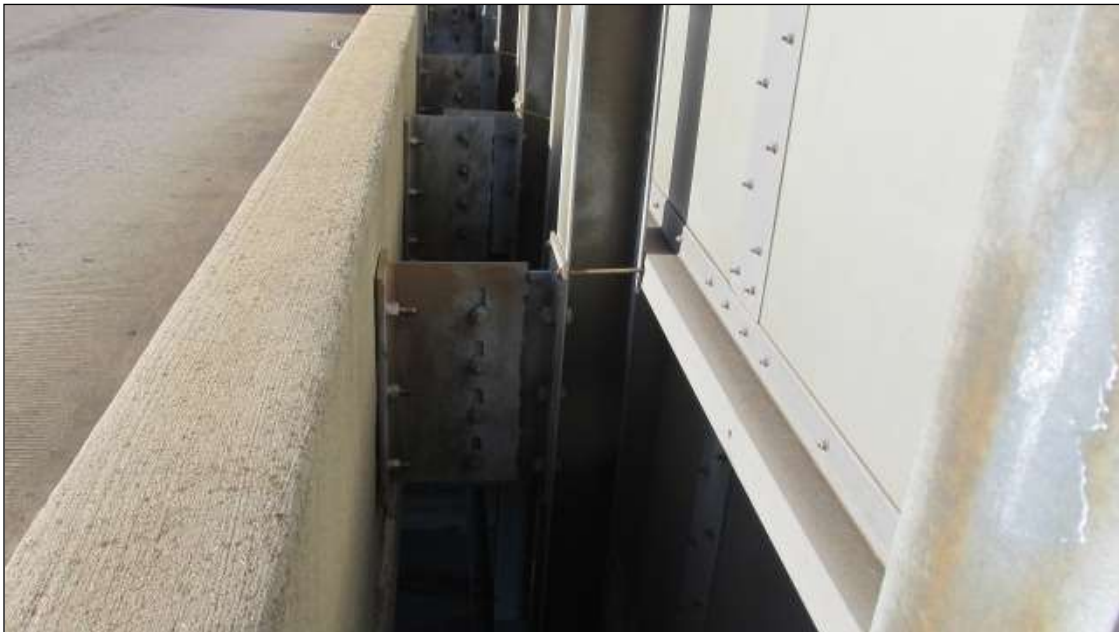
SIGN ATTACHED TO THE RT. RAIL IN SPAN 2 OVER THE ROADWAY.
