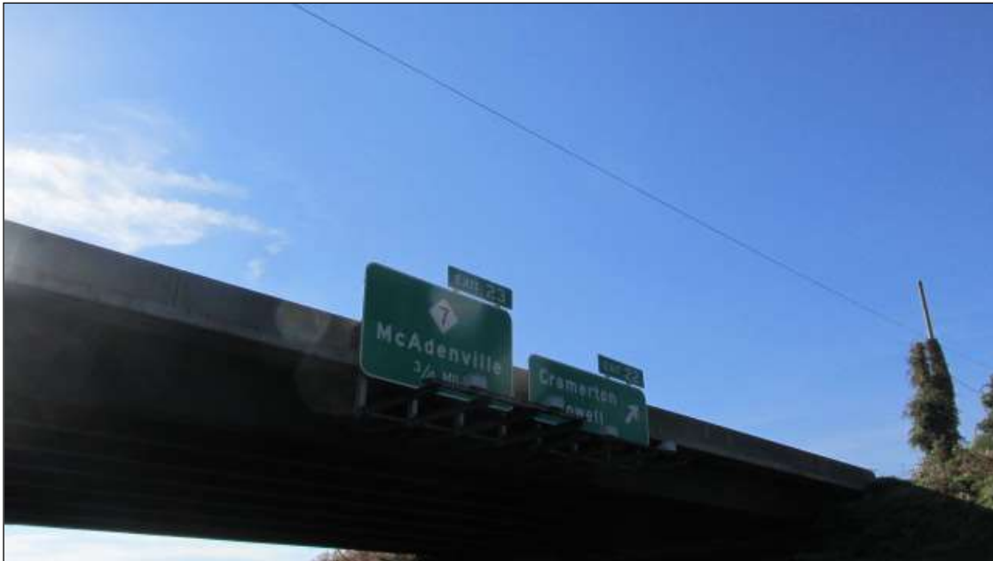
SIGN ATTACHED TIO THE RT, RAIL IN SPAN 2
