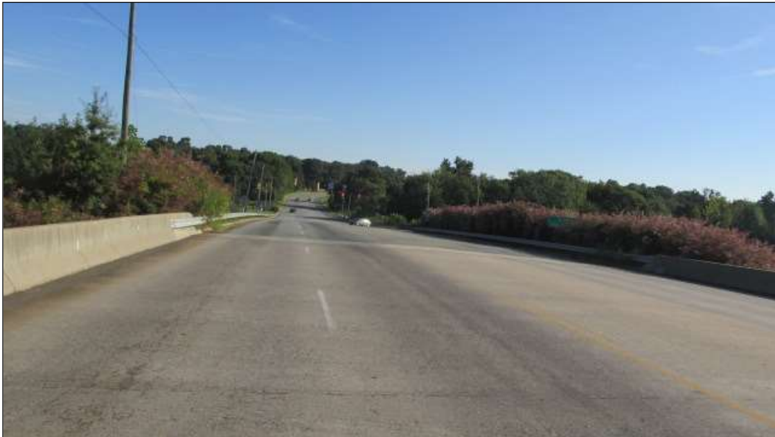
GUARDRAIL LOOKING WEST
