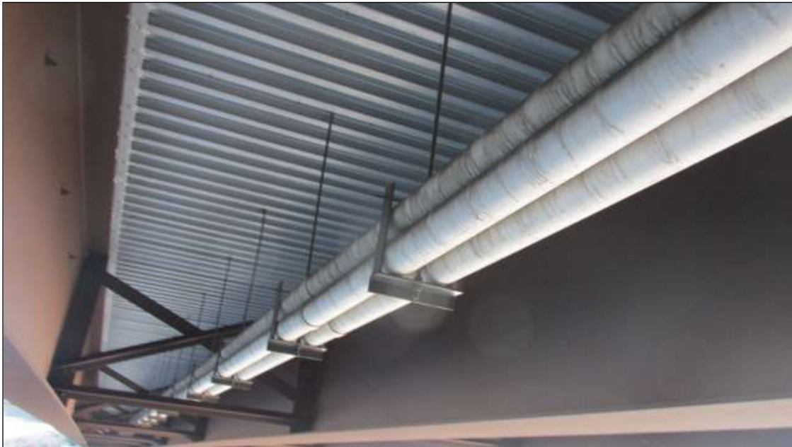
UTILITY IN BAY 7
