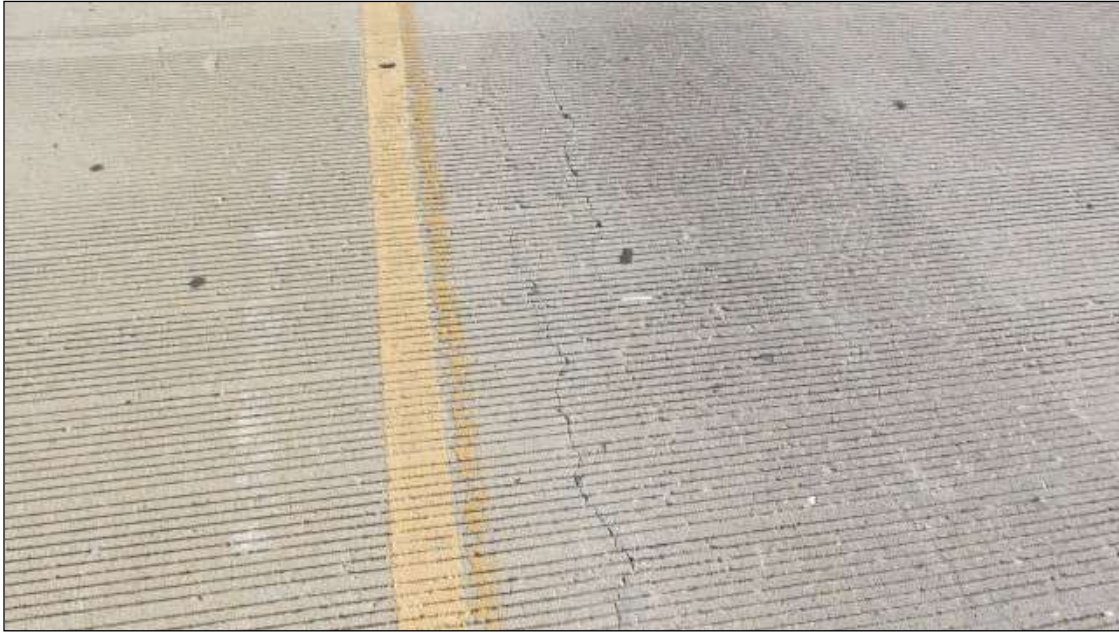
APPROACH SLABS HAVE LONG. CRACKING 1/16" TO 1/8" WIDE FOR FULL LENGTH OF THE SLABS.
